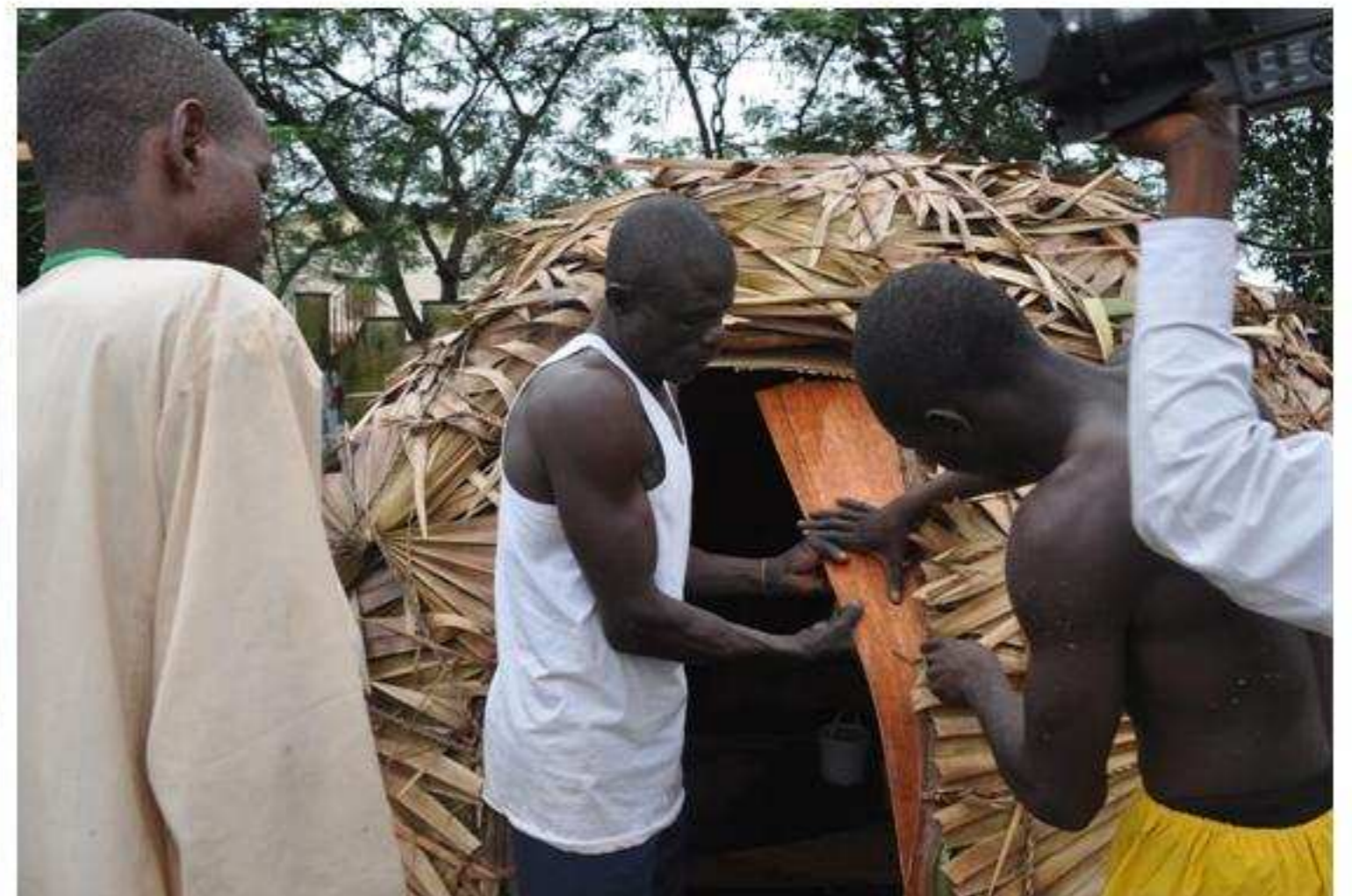
• Construction in progress – Traditional Furnished Apartment– Gombe State
